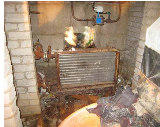
Meter for hot water
