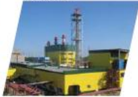
INDUSTRIAL PARK RODNIKI, TAMBOV REGION
