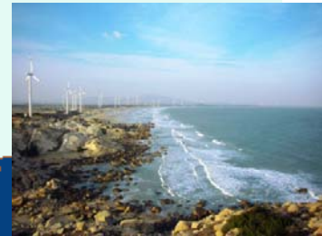
Fujian Zhangpu Liua Wind Power Project. Fujian province, China
